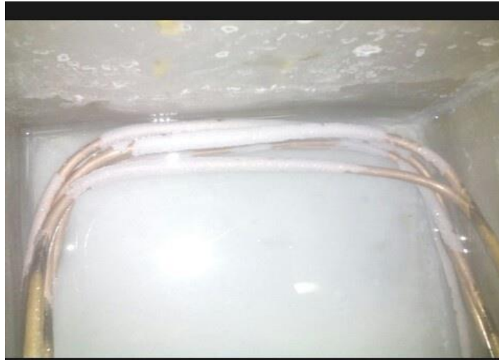
Figure 7 Freezing of pcm in evaporator
