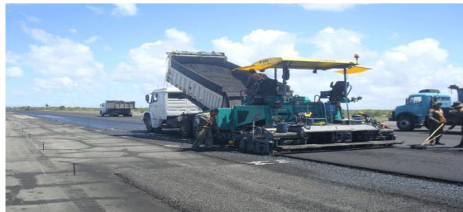
Fig-1.3A- Airport Constructions Bitumen Laying work
