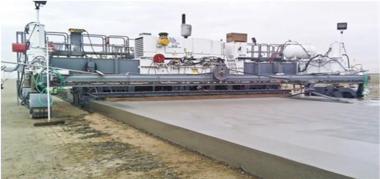
Fig-1.4 -Final working Photo of Active Runway
