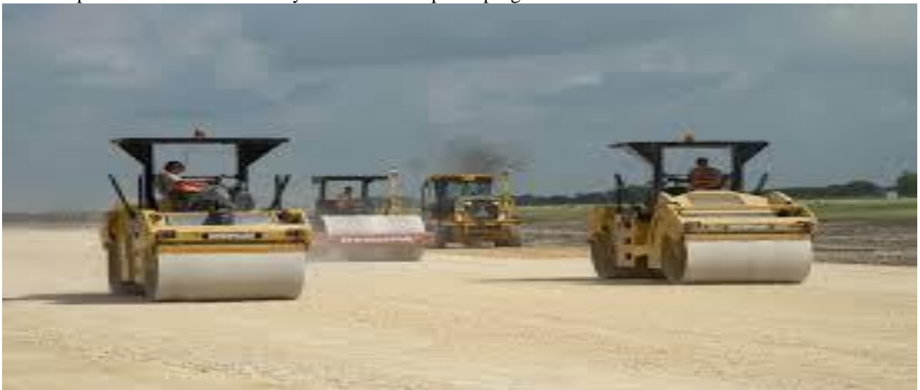
Fig-1.1- Actual Compaction work active runway construction work for WMM layer
